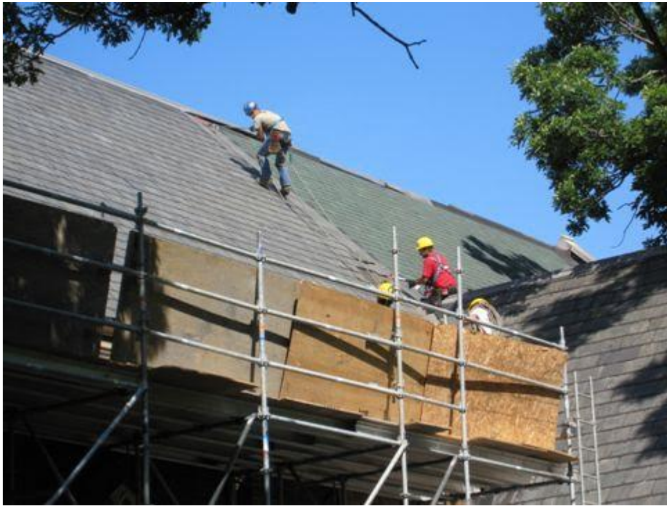
The new roof on the church is coming along quickly!
